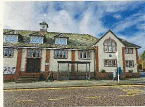
East facing Elevation (north end)
