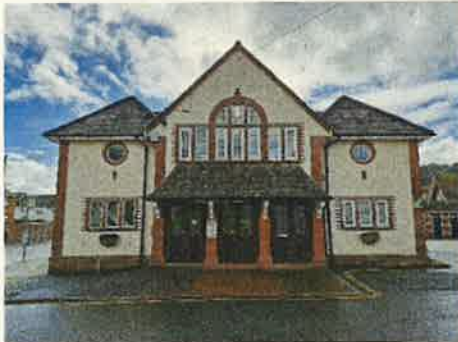
North facing Elevation (main entrance)
