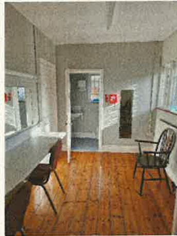
Dressing Room (SE Corner)
