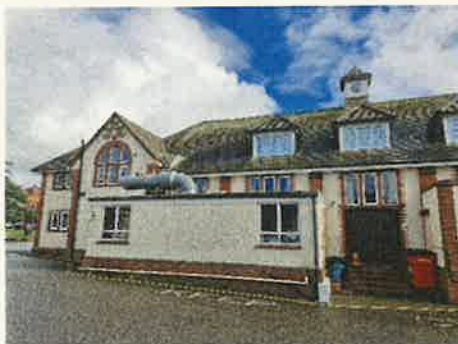
West facing Elevation (north end)
