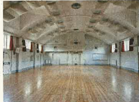
Main Hall (Entrance)
